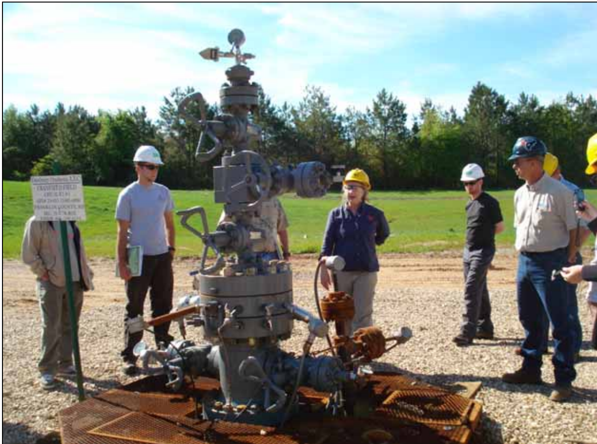
Monitoring/Observation Well (CFU 31-F2 #1), located at the SECARB Phase III Detailed Area of Study in Cranfield, Mississippi. Note the various tools on the well, indicating the multiple MVA tools being deployed at the site.
